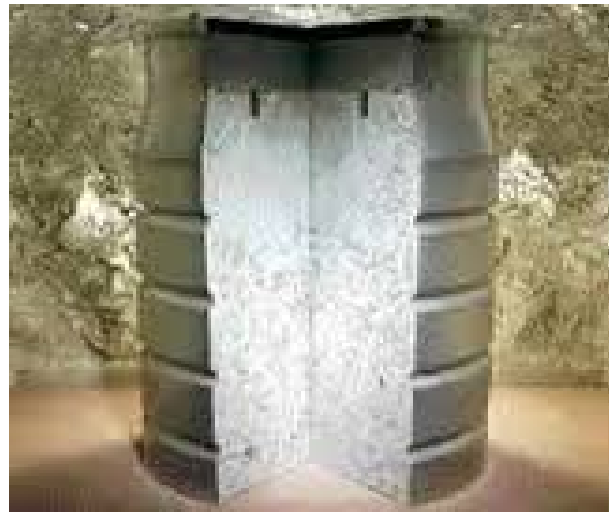
Encased in Concrete
